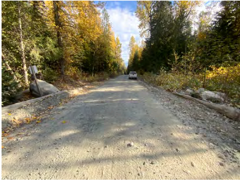
Approach from Left Bank when facing downstream
