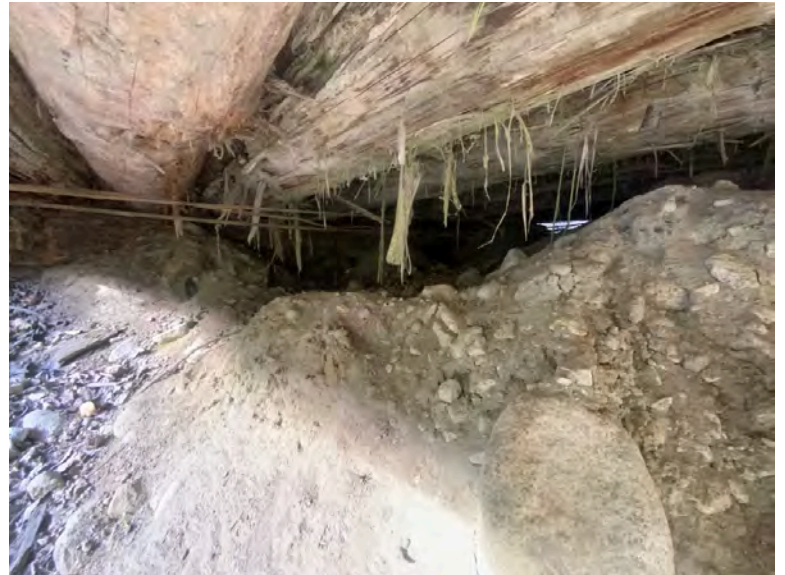
Right Bank Abutment when facing downstream
