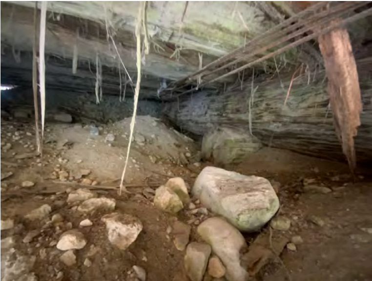
Left Bank Abutment when facing downstream
